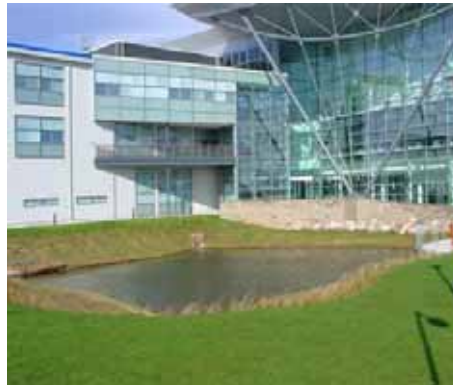
Photo crown copyright. Two balancing ponds at the Met Office Building.
