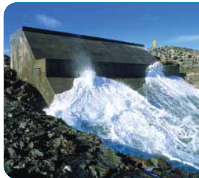
The world's first commercial-scale wave power station, Limpet 500.
